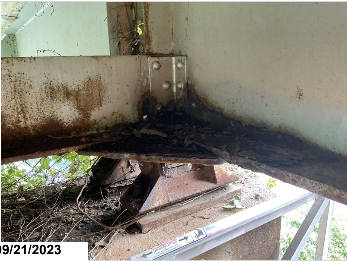
Rust with pack rust & s/l to diaphragm, bottom flange & connecting plate @ Girder 2 @ end of Span 2.(#3)
