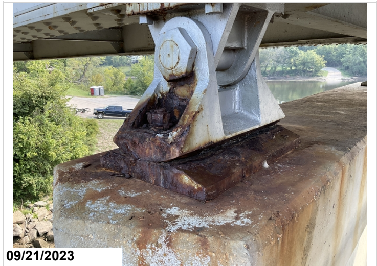
Rust with pack rust to Moveable Bearing 1 @ Bent 4.(#3) (typical)
