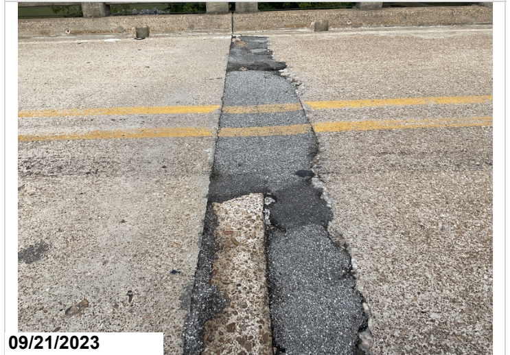
Spalls/patched areas to deck @ beginning of Span 4.(#3)
