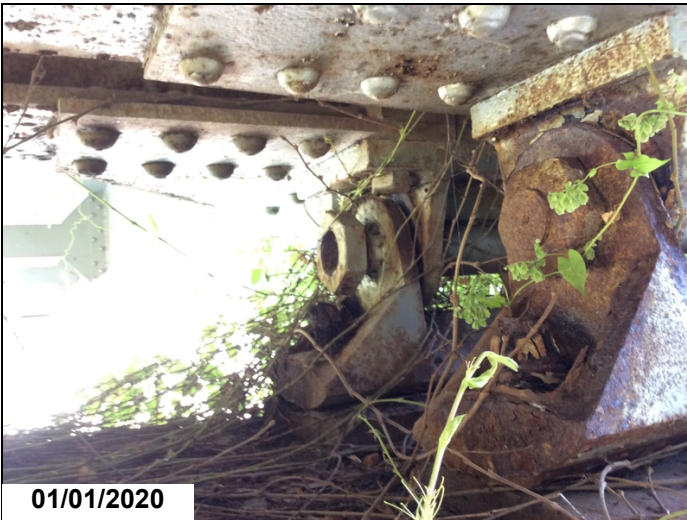
Interior nut has backed off of pin at the ahead side Bearing 2 at Bent 2.
