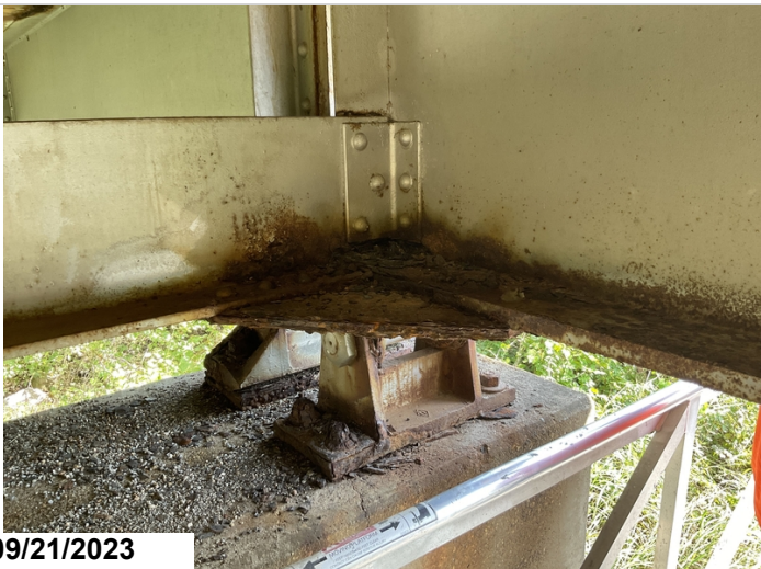
Rust with pack rust & s/l to diaphragm, bottom flange & connecting plate @ Girder 2 @ end of Span 6.(#3)
