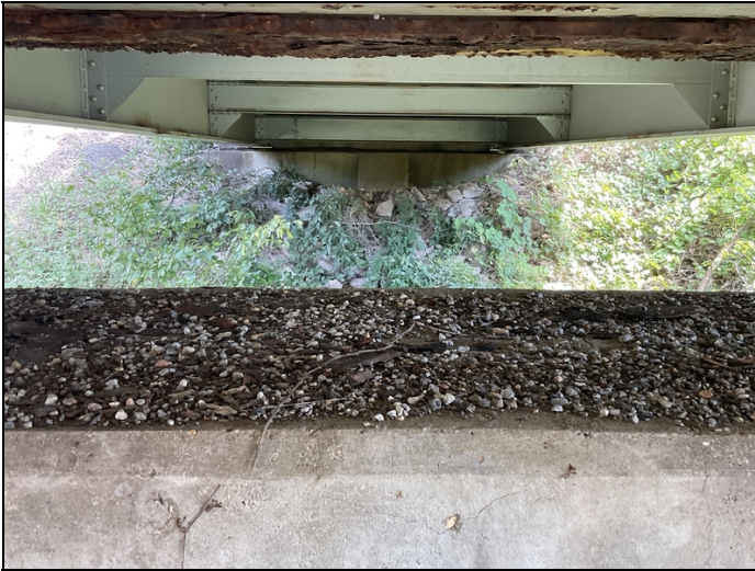
Debris on cap @ Bent 6 & Abutment 2.
