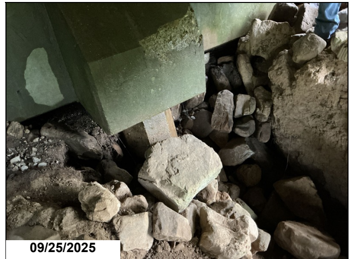
Scour at abutment 1 exposing concrete pile.
