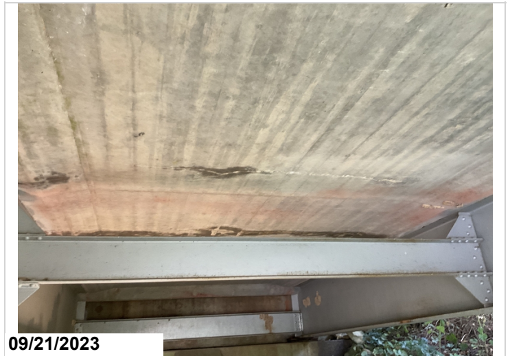
Efflorescent cracking to soffit @ Span 1.(#2)(typical)
