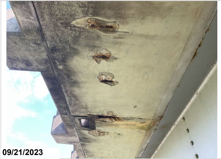
Typical spalls with rebar exposed to overhangs.(#3)(Left overhang @ Span 3)
