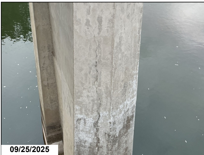
Vertical crack to column 2 at bent 3.
