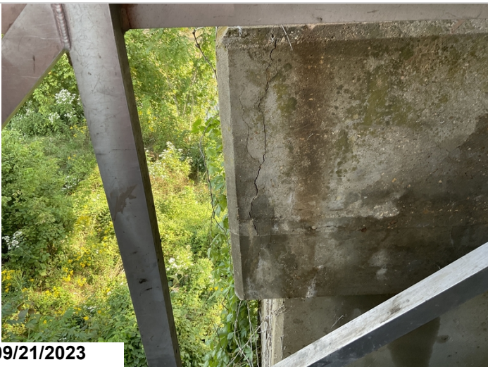
Vertical cracking to Left end of cap a Bent 1.(#3)
