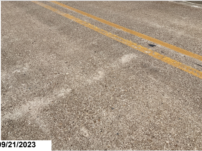
Typical abrasion to deck.(#2)
