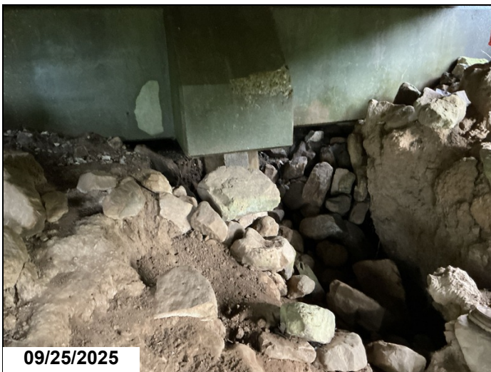
Scour at abutment 1 exposing concrete pile.
