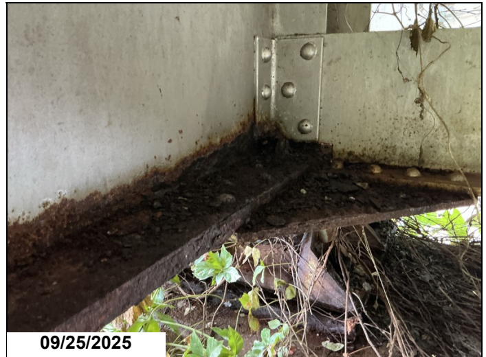
Rust with section loss to girder 1 end of span 2.
