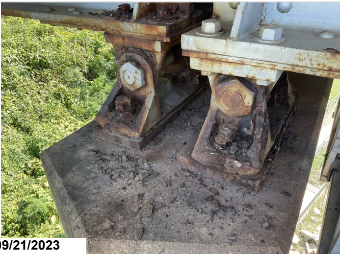
Exterior nuts on rocker pins @ Moveable Bearing 1 on ahead & back sides of Bent 5 have cracks.(#3)
