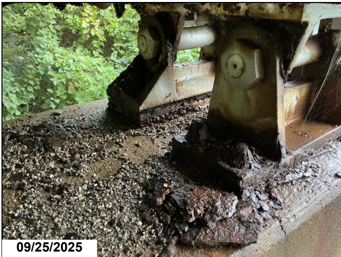
Rust with heavy section loss to anchor bolt nuts to bearing 2 on back and ahead side of bent 6.
