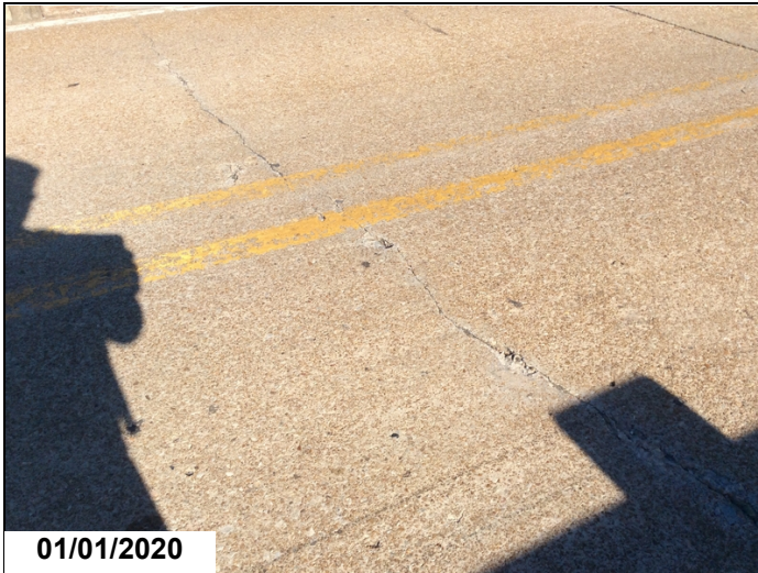
Span 5 Deck cracks and spalls.
