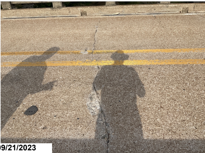
Typical transverse cracking & spalling to deck.(#3)(typical)
