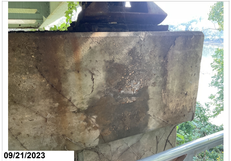
Delaminated areas to Right end of cap @ Bent 1.(#3)
