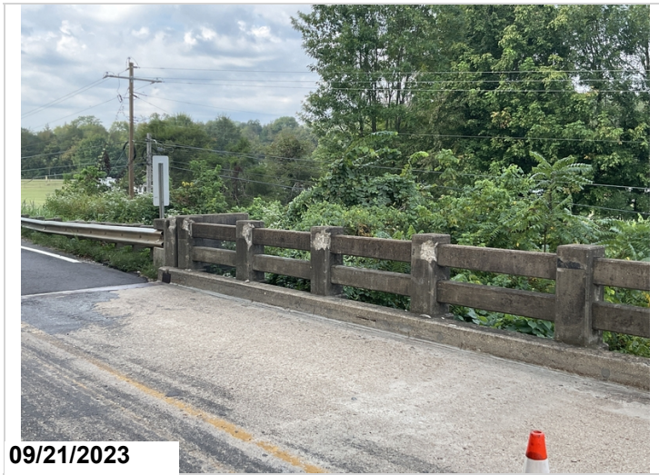
Typical spalling to concrete bridge rail posts.
