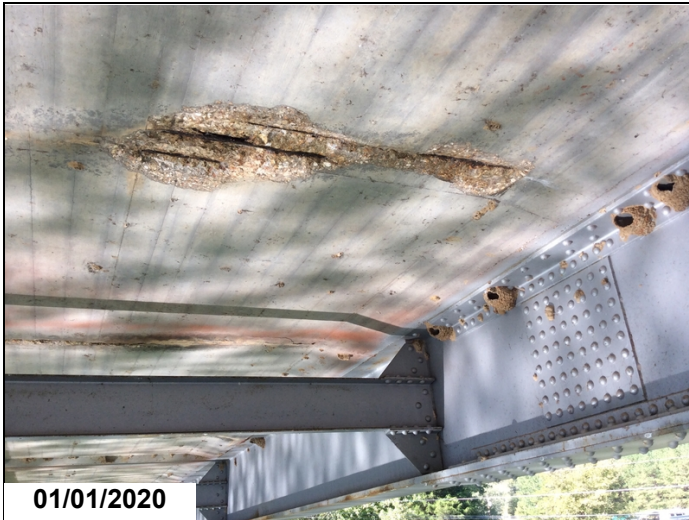
Span 3, Typical spall with exposed rebar to soffit.
