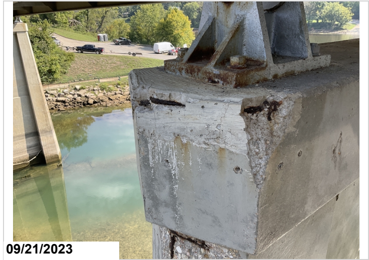
Spall with rebar exposed with s/l to Left end of cap @ Bent 3.(#3)
