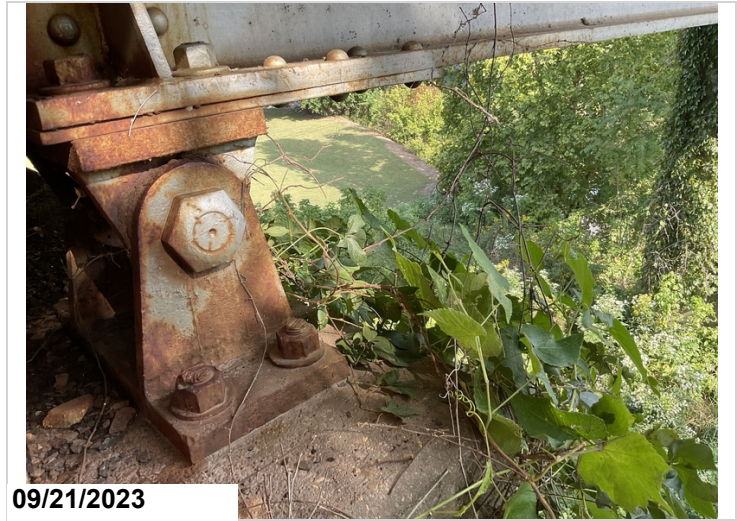
Typical rust to Fixed Bearings.(#2 Bent 1)
