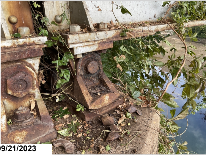
Exterior nut on rocker pin @ Moveable Bearing 2 on ahead side of Bent 2 is missing & Anchor bolt is also missing due to heavy corrosion.(#4)
