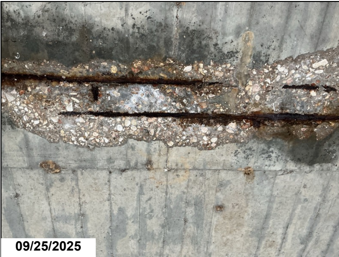
Spall with exposed rebar to undersurface of span 5.
