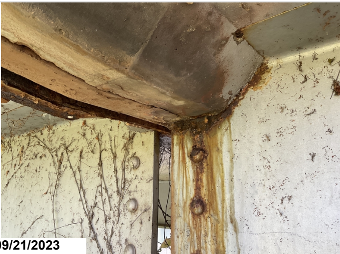
Rust with 5/16" s/l to web below haunch @ Girder 1 @ end of Span 2.(#3)
