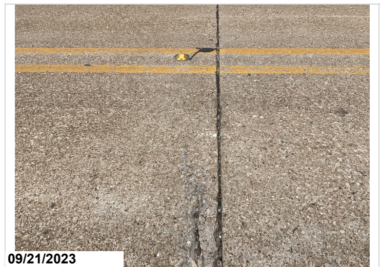
Pourable joint seal is losing adhesion @ Span 5.(#3)
