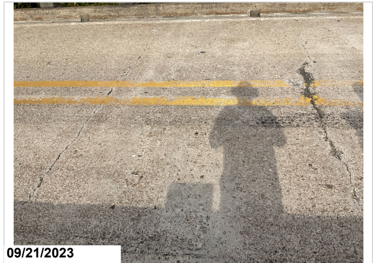
Transverse cracking to deck @ Span 3.(#3)(typical)
