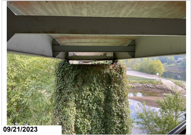
Typical paint condition of girders.
