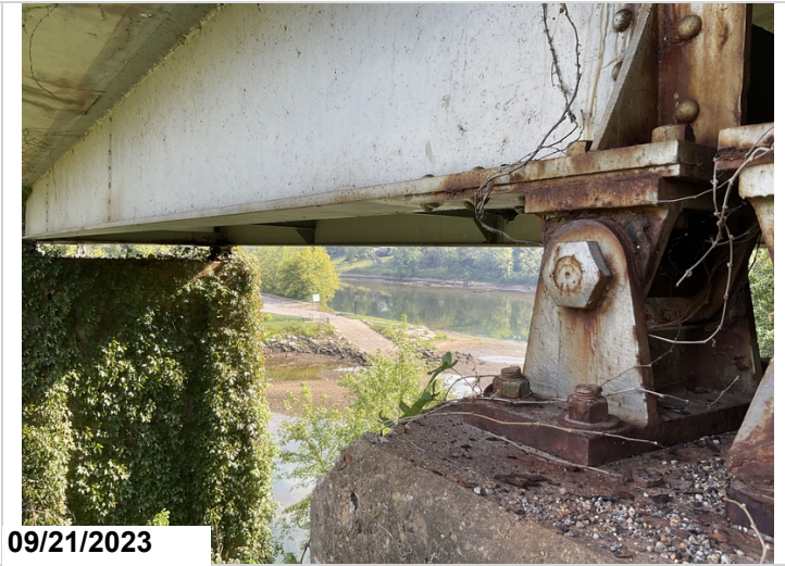
Rust with pack rust to Fixed Bearing 1 @ Bent 1.(#3)
