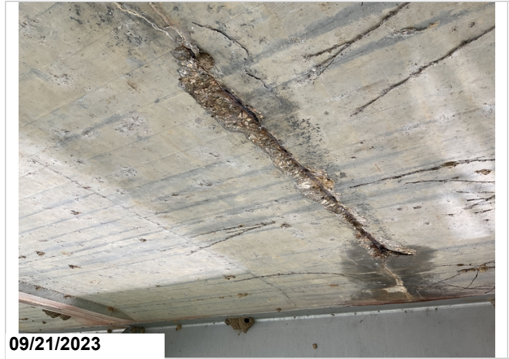
Spalls with rebar exposed with s/l to soffit @ Span 3.(#3) (typical)
