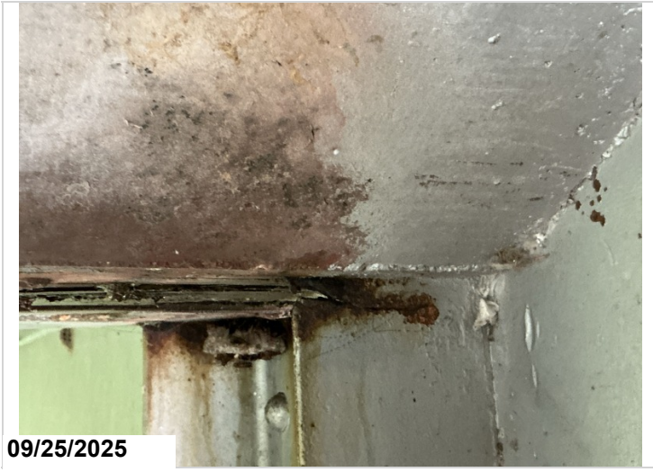
Crack to stiffener on girder 2 end of span 6.
