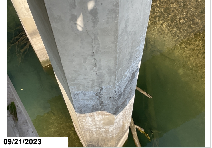
Vertical cracking to Column 2 @ Bent 3.(#2)
