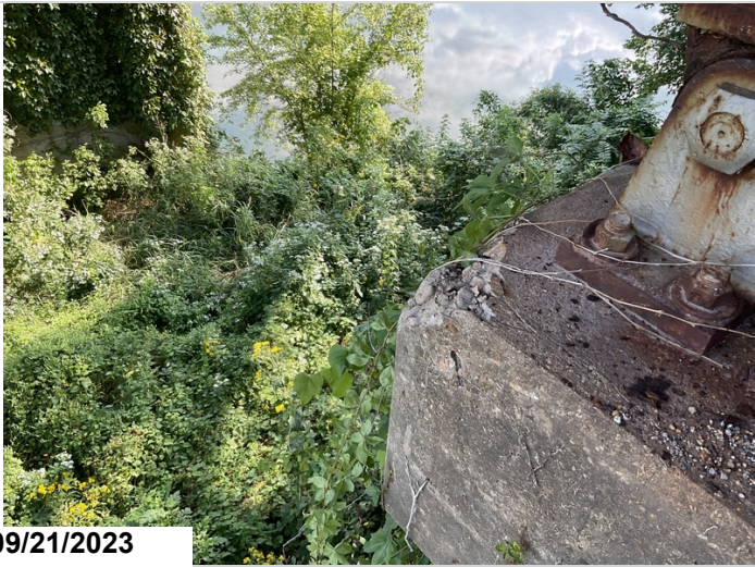
Spall to Left end of cap @ Bent 1.(#3)
