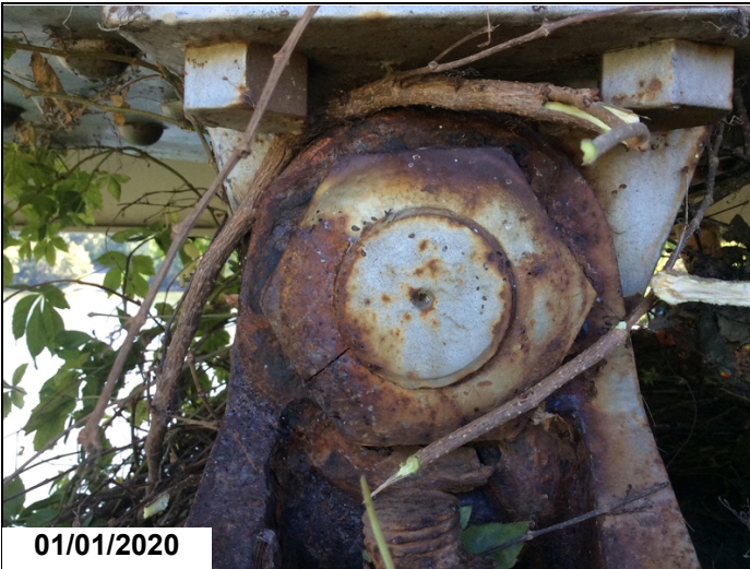
Exterior anchor bolt nut is cracked @ Girder 1 Bent 2 ahead.
