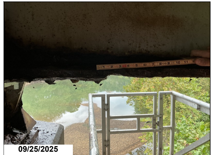
Rust with section loss to girder 1 beginning of span 6.
