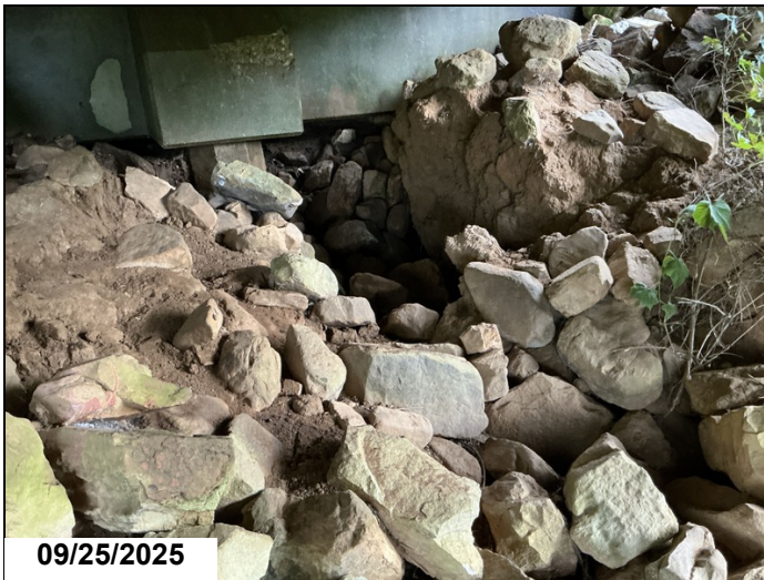
Scour at abutment 1 exposing concrete pile.
