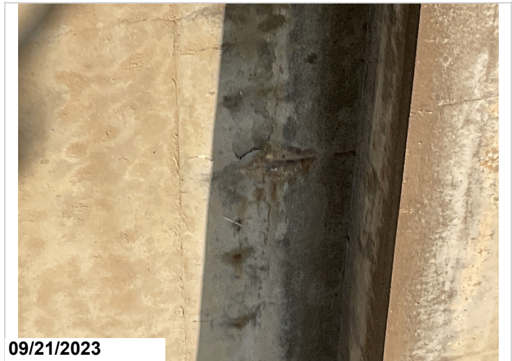
Spall with rebar exposed with s/l to Concrete Pier Wall @ Bent 5.(#3)
