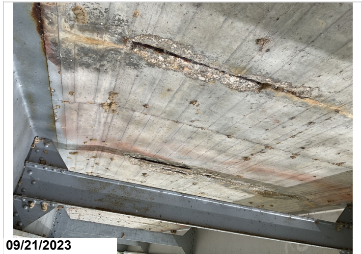
Spalls with rebar exposed with s/l to soffit @ Span 4.(#3) (typical)
