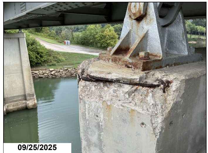
Spall with exposed rebar to left end of cap at bent 3.
