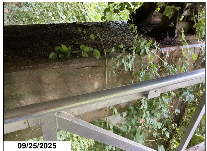
Horizontal crack to ahead side of cap at bent 1.
