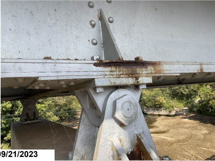
Rust with pack rust between cover plate & bottom flange @ Girder 2 @ end of Span 3.(#3)
