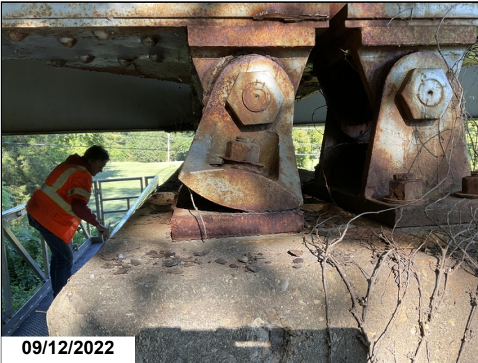
Rocker bearings at Bent 1 have rotated ahead closing deck joint.
