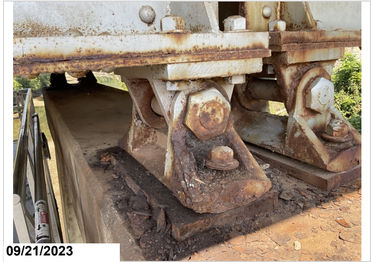
Exterior nut on rocker pin @ Moveable Bearing 2 @ backside of Bent 5 is cracked.(#3)
