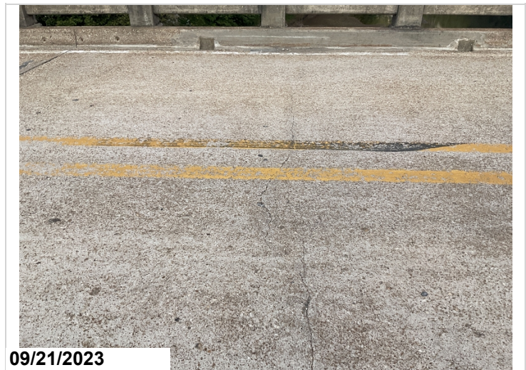
Typical transverse cracking to deck.(#3)(typical)
