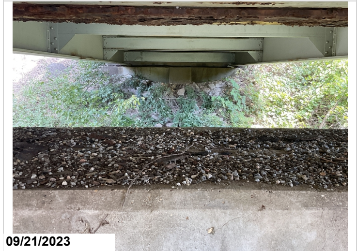
Debris on cap @ Bent 6 & Abutment 2.
