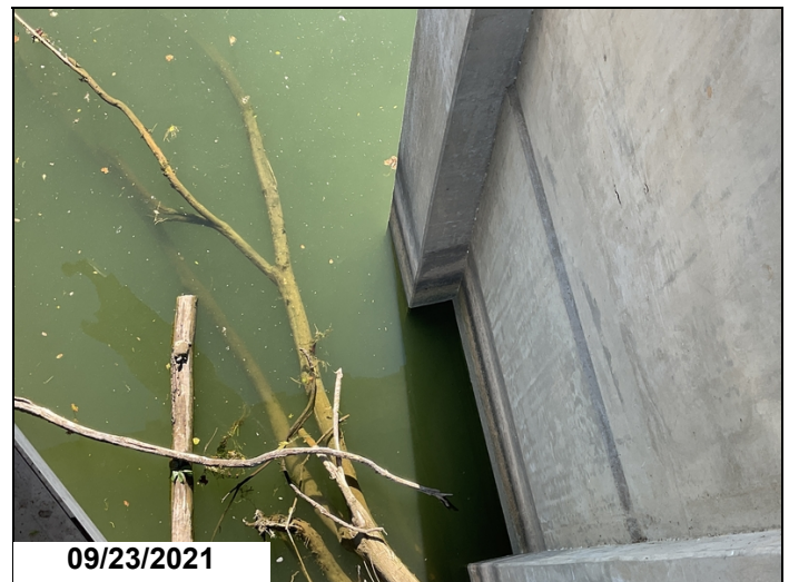
Channel has minor scour with tops of footings exposed at Bents 3 thru 5.
