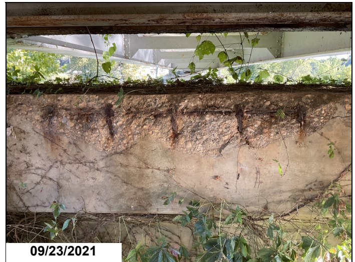
Caps and columns at Bents 1 thru 5. Spalls with rebar exposed and delaminated areas. Backside of bent 2.
