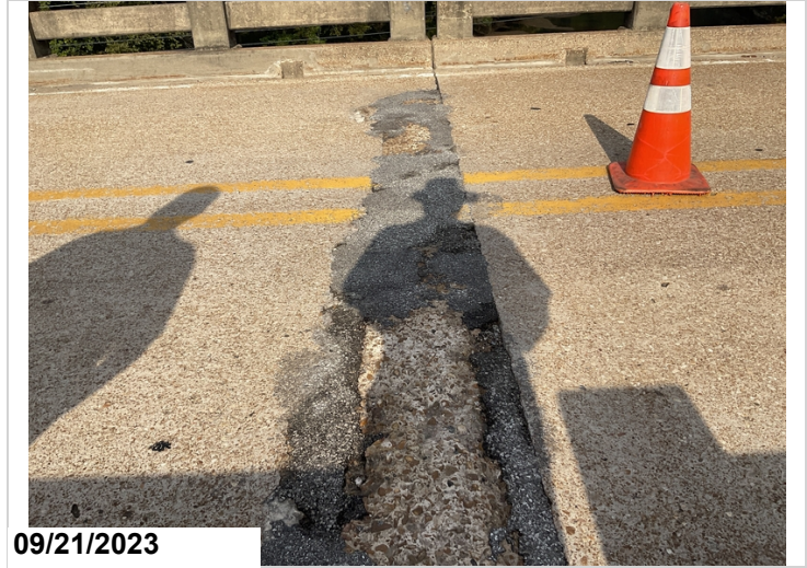
Spalls/patched areas to deck @ end of Span 4.(#3)
