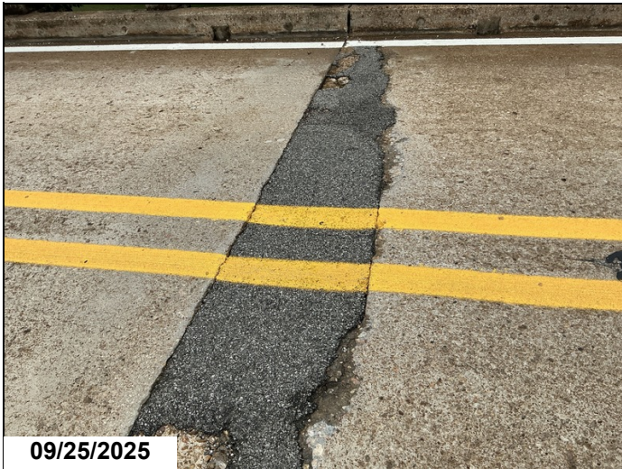
Deep spalls and delaminated areas to deck with some exposed rebar.(covered with asphalt).
