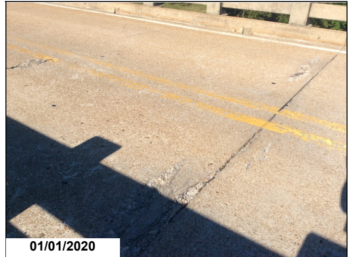
Spalls to deck at Span 4.
