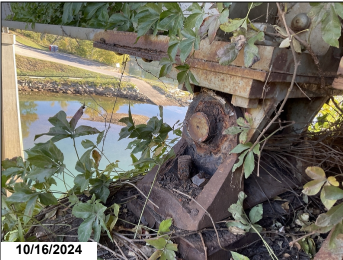
Bent 2, ahead, bearing 1: is missing the exterior nut.
