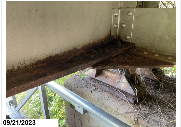
Rust with pack rust with s/l to bottom flange & connecting plate @ Girder 1 @ end of Span 2.(#3)
