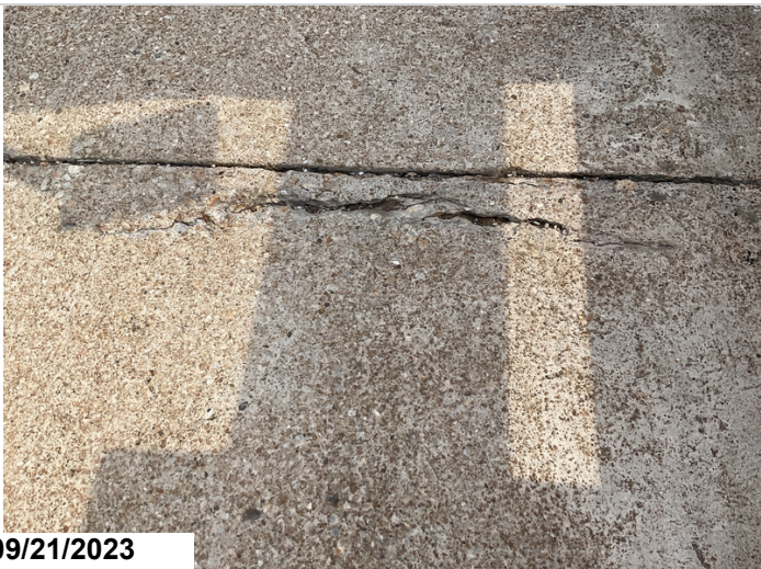
Spalls to deck @ Span 5.(#3)
