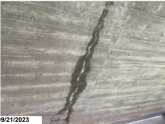
Efflorescent cracking to soffit @ Span 2.(#2)(typical)
