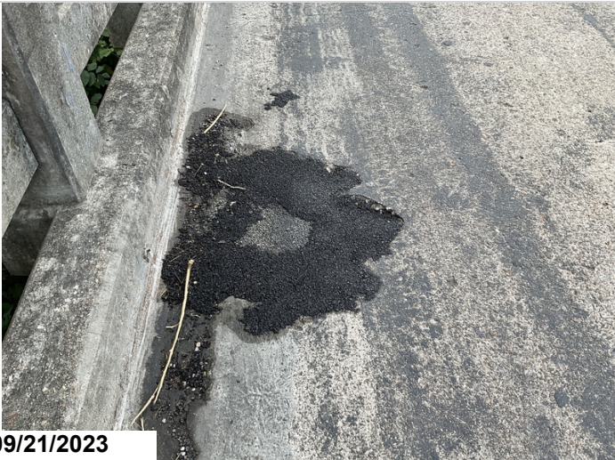
Patched area to deck @ Span 1.(#2)
