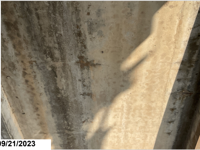
Horizontal cracking to Concrete Pier Wall @ Bent 5.(#2)
