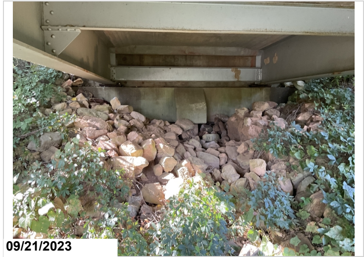
Erosion to slope exposing 1 pile @ Abutment 1.(#3)
