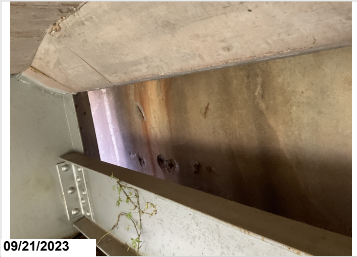
Spalls with rebar exposed to Abutment 2.(#3)
