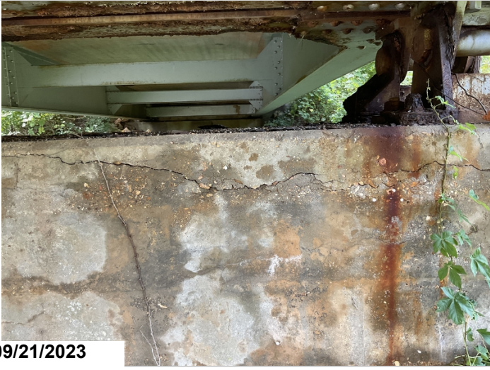
Horizontal cracking to ahead of cap @ Bent 1.(#3)
