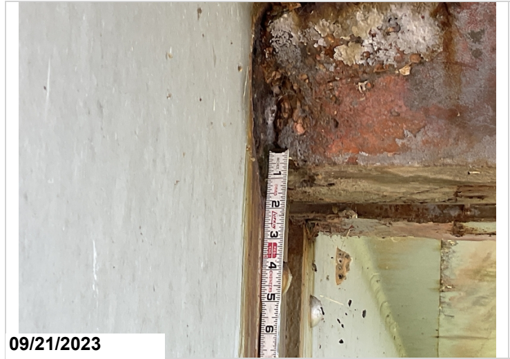
Rust with 1/2" s/l to web below haunch @ Girder 2 @ end of Span 6.(#3)
