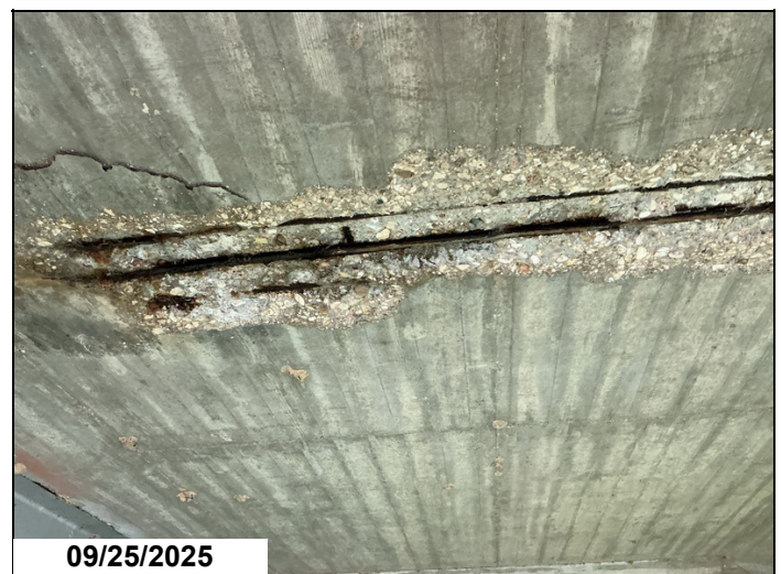
Spall with exposed rebar to undersurface of span 6.
