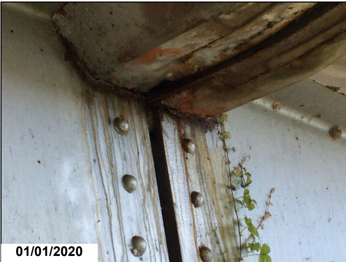
Rust to haunch area of Girder 2 at Bent 1.
