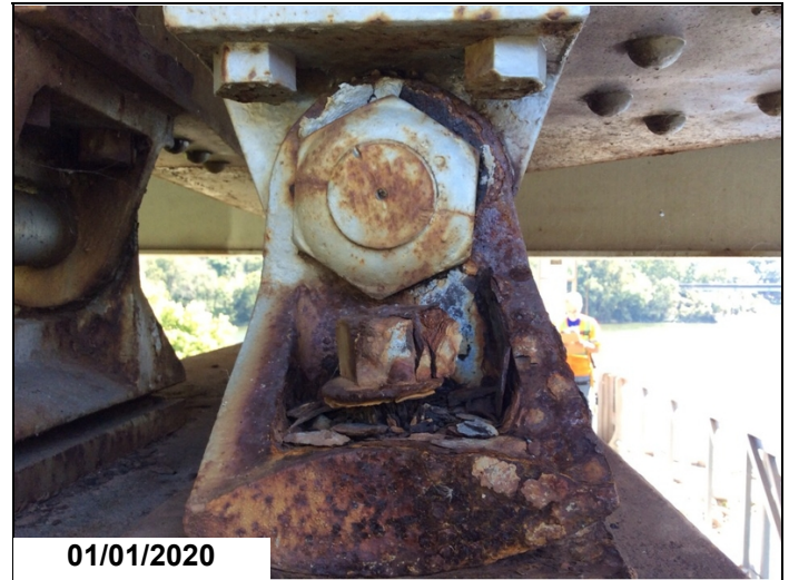
Section loss to anchor bolt & cracked nut @ Girder 1 Bent 5.
