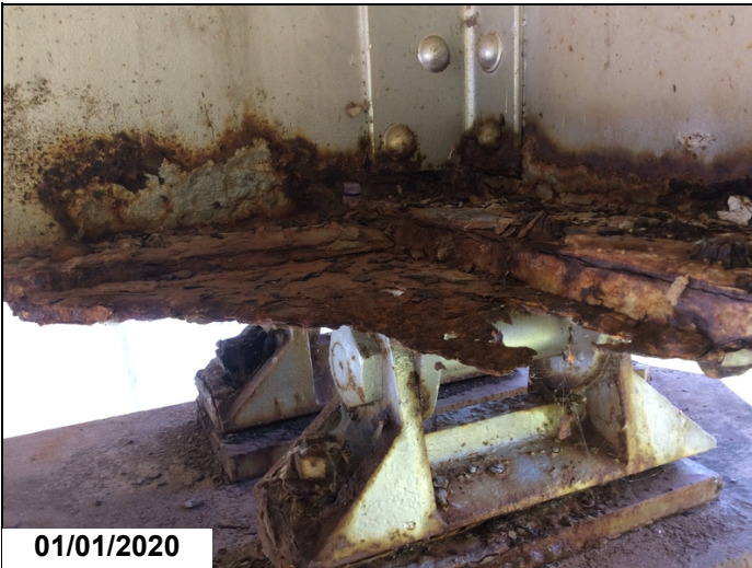
Diaphragm connection plate at Girder 1, Bent 5 ahead side.
