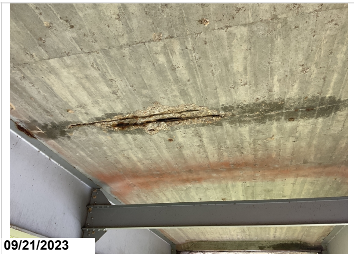
Spalls with rebar exposed with s/l to soffit @ Span 2.(#3) (typical)
