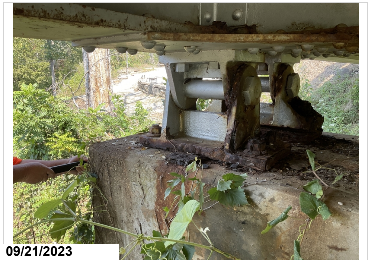
Rust with pack rust to Fixed Bearing 1 @ Bent 7.(#3)
