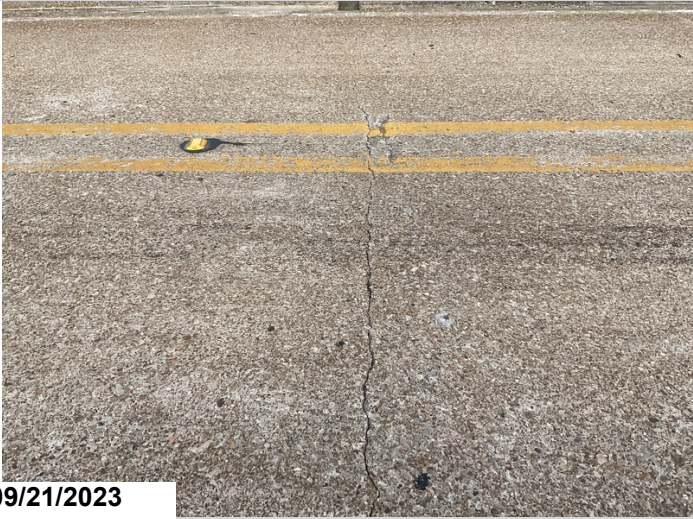
Typical transverse cracking to deck.(#3)
