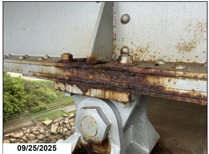
Rust with pack rust and section loss to girder 1 over bent 4.
