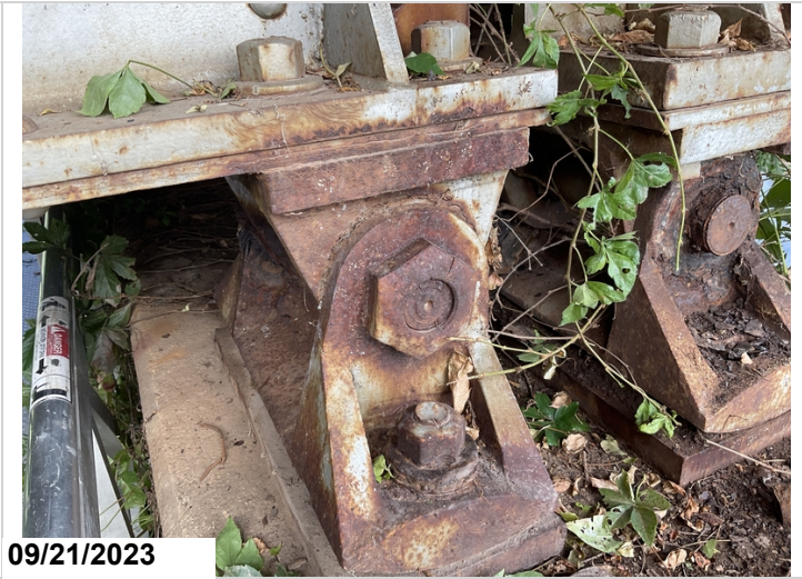
Exterior nut on rocker pin @ Moveable Bearing 2 @ backside of Bent 2 is cracked.(#3)
