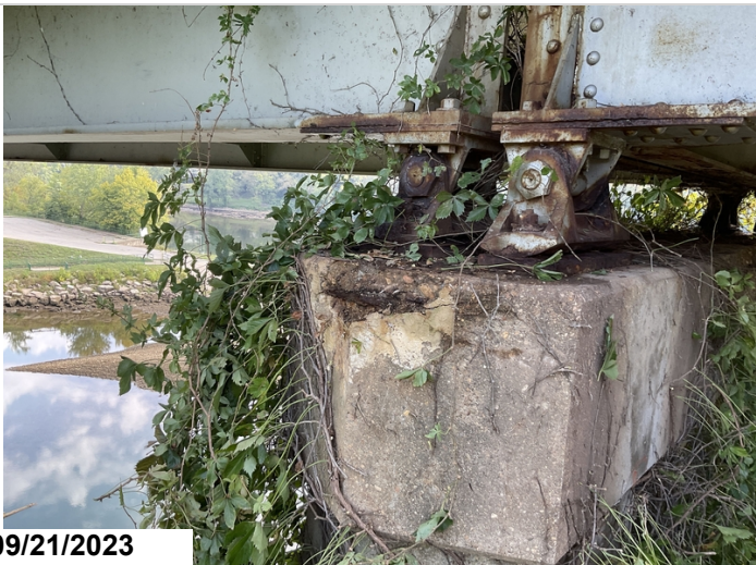
Spall with rebar exposed with s/l to Left end of cap @ Bent 2.(#3)
