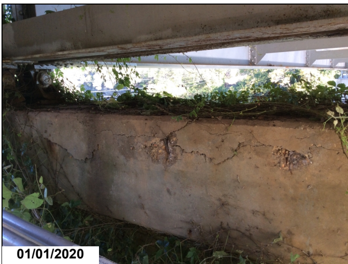
Large delaminated area, Spalls with exposed rebar at Bent 2 back side of cap.
