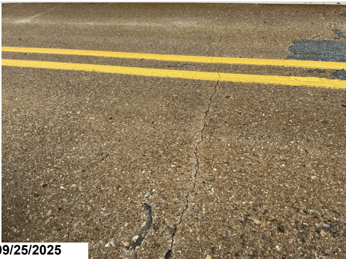
Transverse cracks to deck at all spans.
