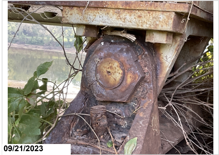
Exterior nut on rocker pin @ Moveable Bearing 1 on ahead side of Bent 2 has 2 cracks.(#3) Anchor bolt nut is also missing due to heavy corrosion.(#3)
