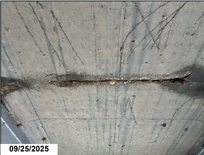
Spall with exposed rebar to undersurface of span 3.
