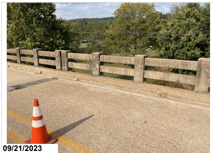
Typical spalling to concrete bridge rail posts.
