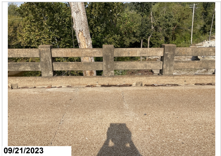
Typical spalls with rebar exposed to concrete bridge rail posts.#2)
