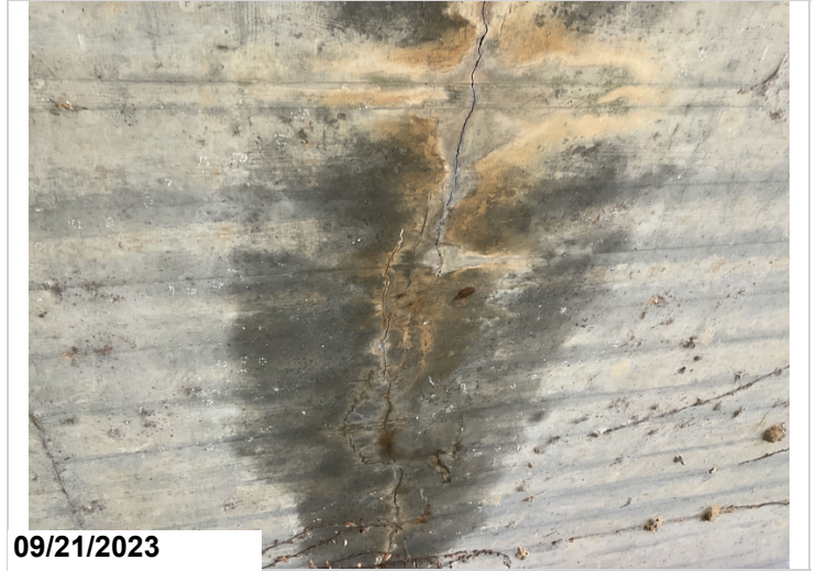
Efflorescent cracking with rust stains to soffit @ Span 3.(#3) (typical)
