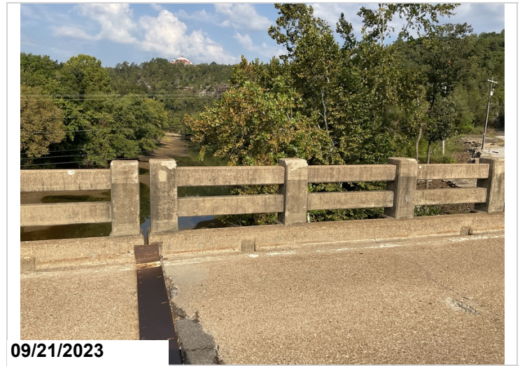
Typical spalling to concrete bridge rail posts.
