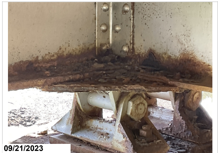
Rust with pack rust & s/l to diaphragm, bottom flange & connecting plate @ Girder 2 @ beginning of Span 6.(#3)
