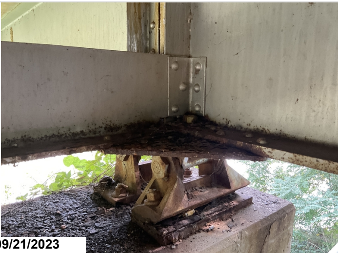
Rust with pack rust & s/l to diaphragm, bottom flange & connecting plate @ Girder 2 @ end of Span 1.(#3)
