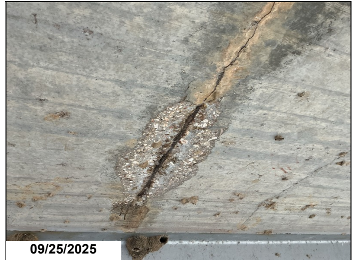
Spall with exposed rebar to undersurface of span 4.
