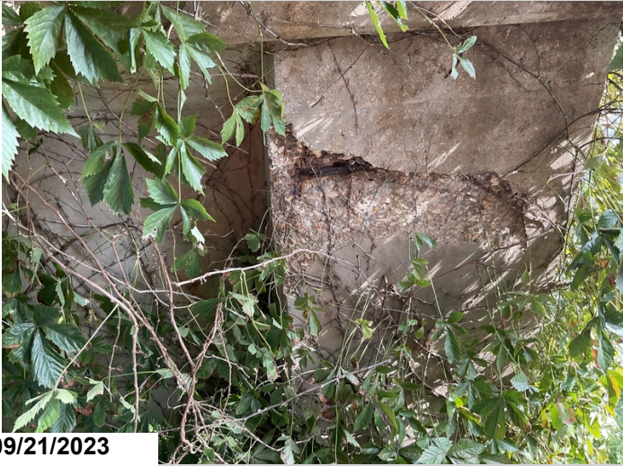
Spalls with rebar exposed with s/l to backside of Column 2 @ Bent 2.(#3)
