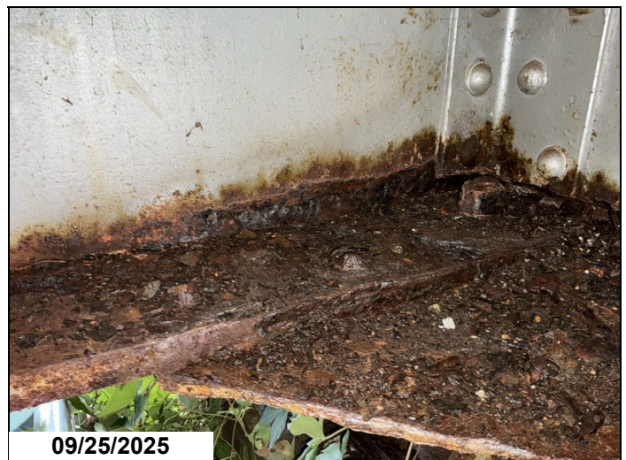
Section loss to bottom of web @ Girder 1 @ end of Span 1.
