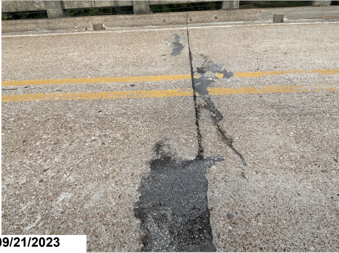
Spalls/patched areas to deck @ end of Span 4.(#3)
