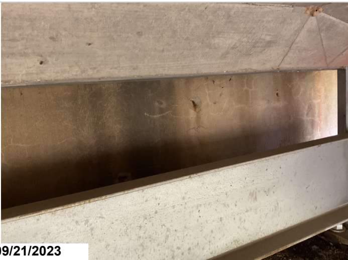
Area of map cracking to Abutment 2.(#2)
