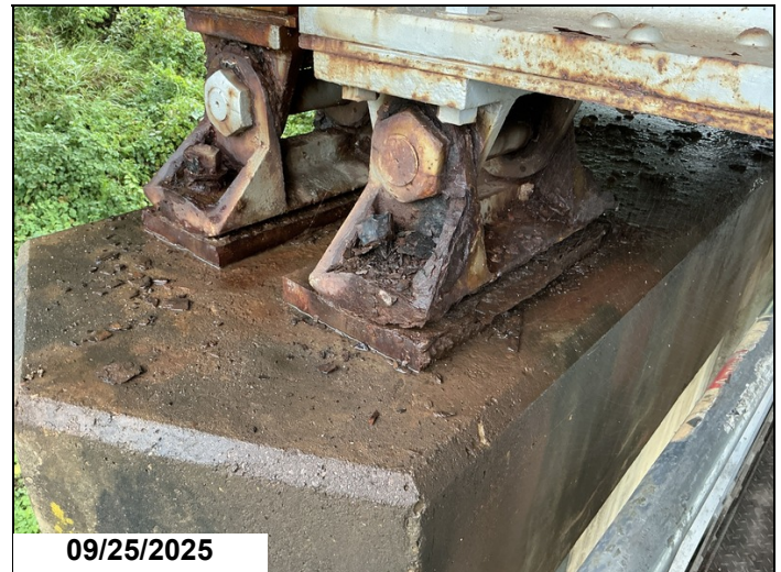
Rust with pack rust and anchor bolt missing to bearing 1 back side of bent 5.
