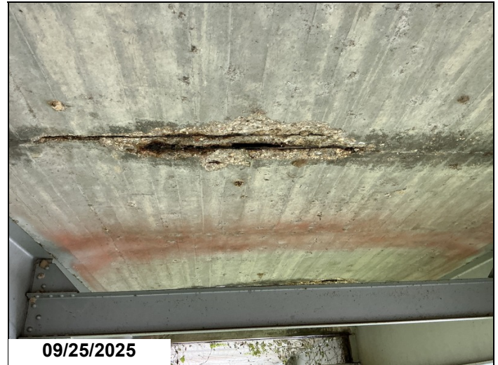
Spall with exposed rebar to undersurface of span 2
