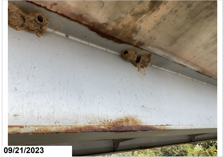
Rust to Girder 2 @ 3rd drain opening @ Span 3.(#3)
