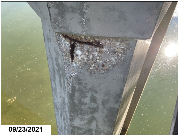
Caps and columns at Bents 1 thru 5. Spalls with rebar exposed and delaminated areas. Column 1 @ bent 3.
