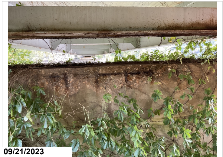
Spalls with rebar exposed with s/l to backside of cap @ Bent 2.(#3)
