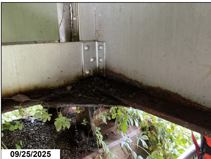
Rust with section loss to girder 1 beginning of span 2.
