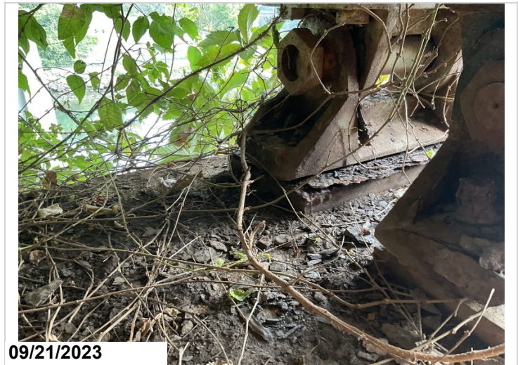
Anchor bolt is missing @ Moveable Bearing 2 on ahead side @ Bent 2.
