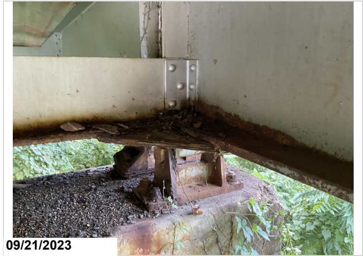
Rust with pack rust & s/l to diaphragm, bottom flange & connecting plate @ Girder 1 @ beginning of Span 2.(#3)
