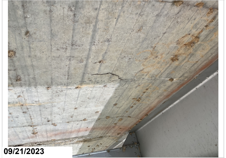
Delaminated area to soffit @ Span 4.
