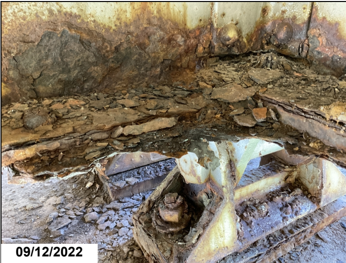
Span 6 - Girder 1 has heavy section loss with part of the gusset plate at bottom flange missing at beginning of span.
