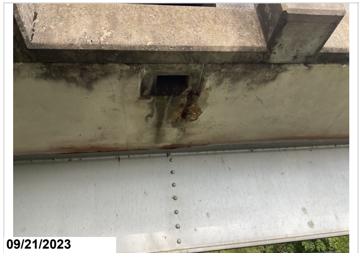
Typical spalls with rebar exposed with s/l to overhangs.(#3)
