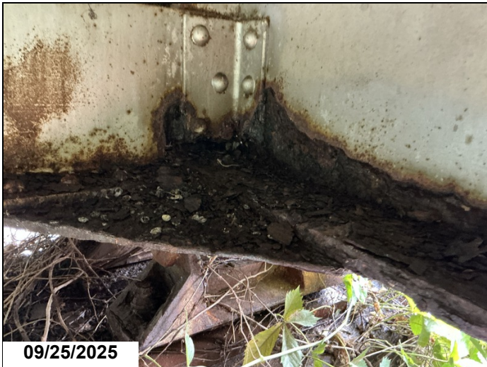
Rust with section loss to girder 2 end of span 2.
