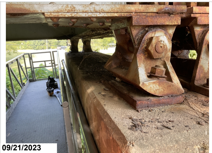
Moveable Bearings @ Bent 1 have rotated ahead to the max.(#4)
