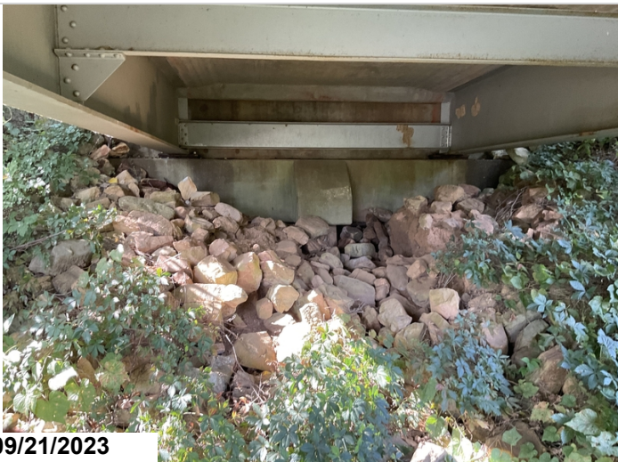
Erosion to slope exposing 1 pile @ Abutment 1.(#3)
