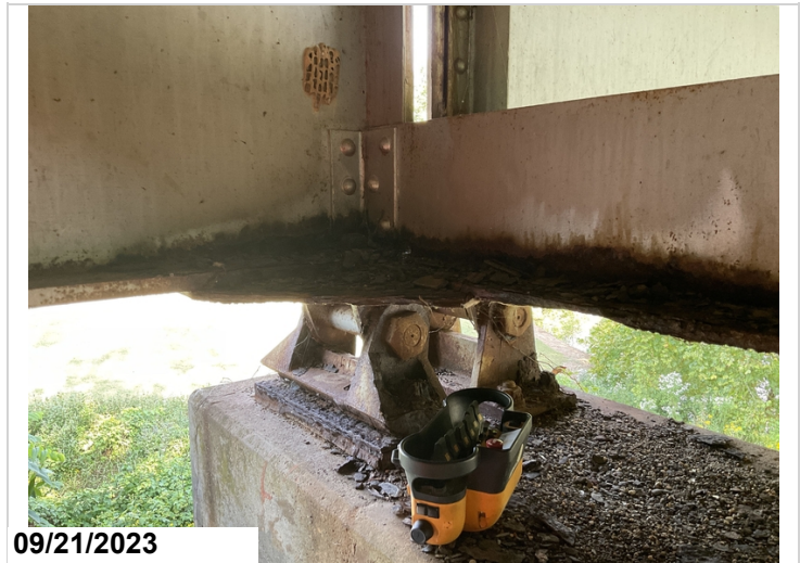
Rust with pack rust & s/l to diaphragm, bottom flange & connecting plate @ Girder 1 @ end of Span 1.(#3)
