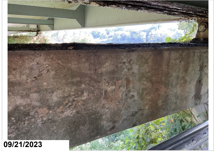
Horizontal cracking to backside of cap @ Bent 1.(#3)
